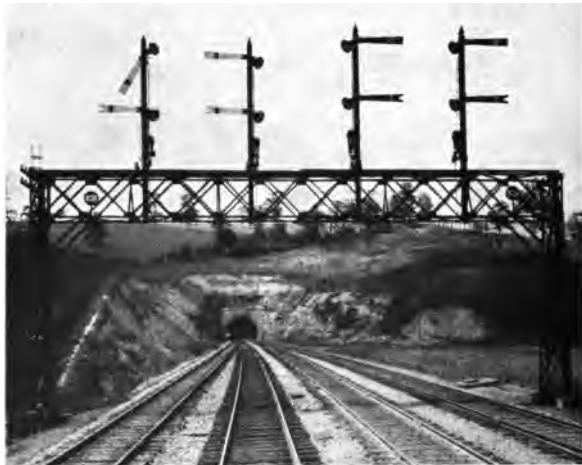
Automatic Block Signals P. R. R.—Westinghouse Electro-Pneumatic
